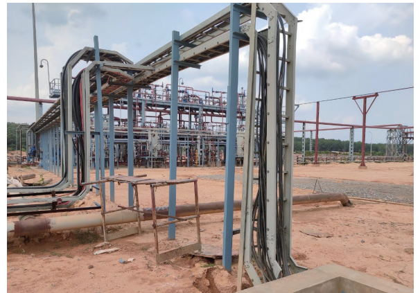
GRP cable ladder at onshore applications
