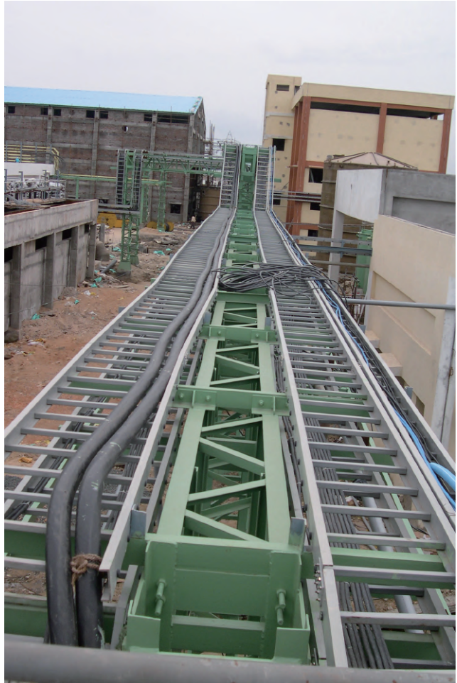
Desalination plant - Chennai
