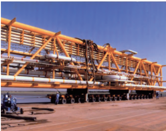
Bridge connecting offshore platforms - 1998
