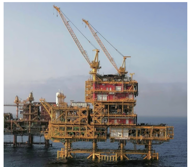
GRP cable ladder and trays on offshore
